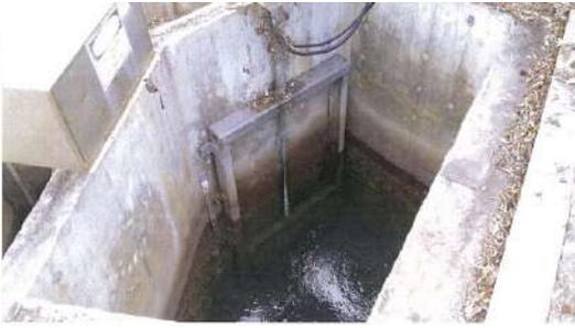
The left photo shows the gate valve mechanism in Joy Beer park that controls water flows between the ocean and the main lake. The right hand photo is the view inside the valve chamber with one of the control valves sitting against the far wall.
