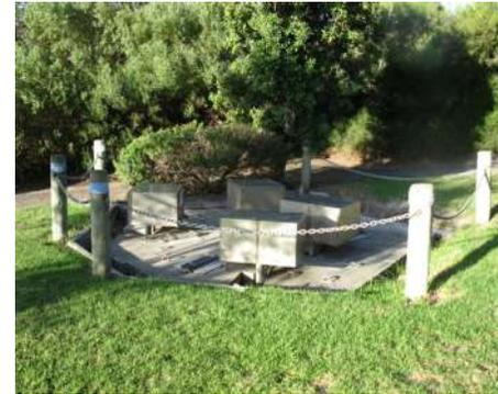
This photo shows the valves that control water flow into and out of Encounter Lakes. The valve mechanisms, after almost 30 years and are expected to be replaced in the 2016/17 financial year.
