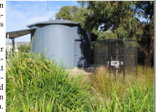
The pump, to the right, transfers water from the main lake to Franklin Island where the water level is a metre higher. At a time of low tide in the sea, water is released from both lakes to lower levels and flush the inlet pipe. Water from Franklin Island provides a stronger flushing action.
